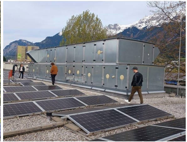
The elementary school Neuarzl in Innsbruck achieved the EnerPHit standard following a retrofit. The advantages are a greatly reduced heating demand and significantly increased thermal comfort for all users in both winter and summer. A large-scale PV system and a ventilation system are installed on the roof. © Passive House Institute
