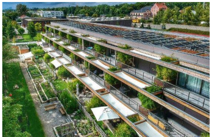
This apartment building in Munich has received Passive House Plus certification. The owners' association operates the photovoltaic system on the roof itself and also convinced the city's public utility company of this model. © StadtNatur
