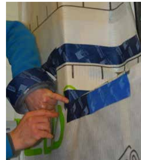
Figure 92: Demonstration in airtightness taping techniques. © MosArt
