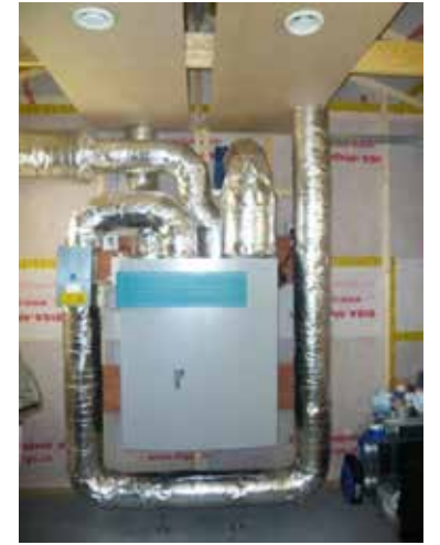
Figure 78: Even for trainees focussed on building fabric, a brief introduction to the critical role of the MVHR system for human health and comfort is integral to the system and training would be very important. © MosArt
