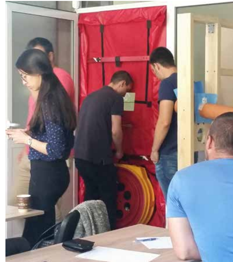
Figure 22: Quality assurance: air tightness testing. © EnEffect
