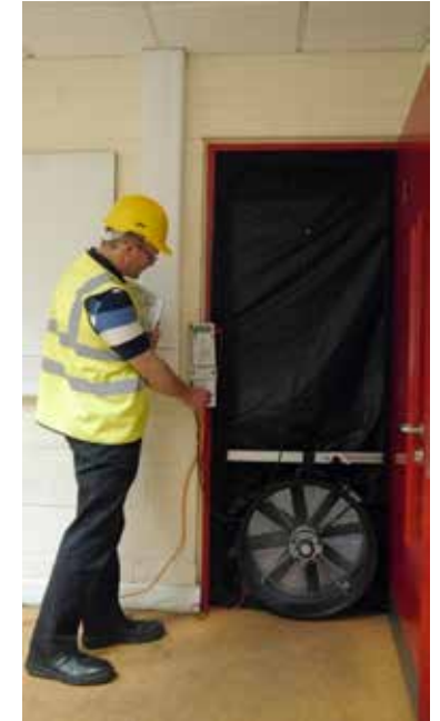
Figure 95: Airtightness testing with fan in door open. © MosArt
