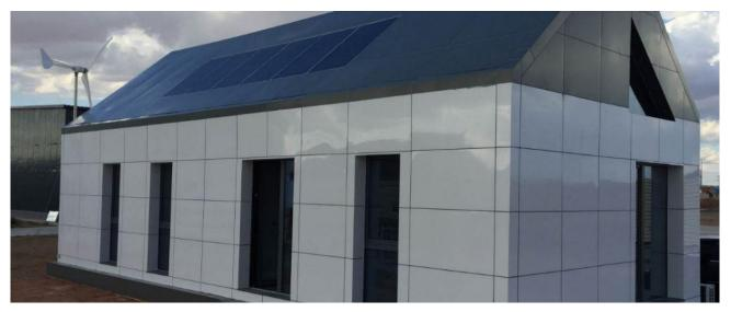
The shipping containers after conversion. The façade of the Passive House pilot project consists of anodised aluminium panels which reflect the countryside. In winter the floor slab can store heat for a long time and helps keep the building pleasantly cool in summer. In Mongolia the rural population will be provided with comfortable housing in order to reduce migration to cities. © Ludwig Rongen
